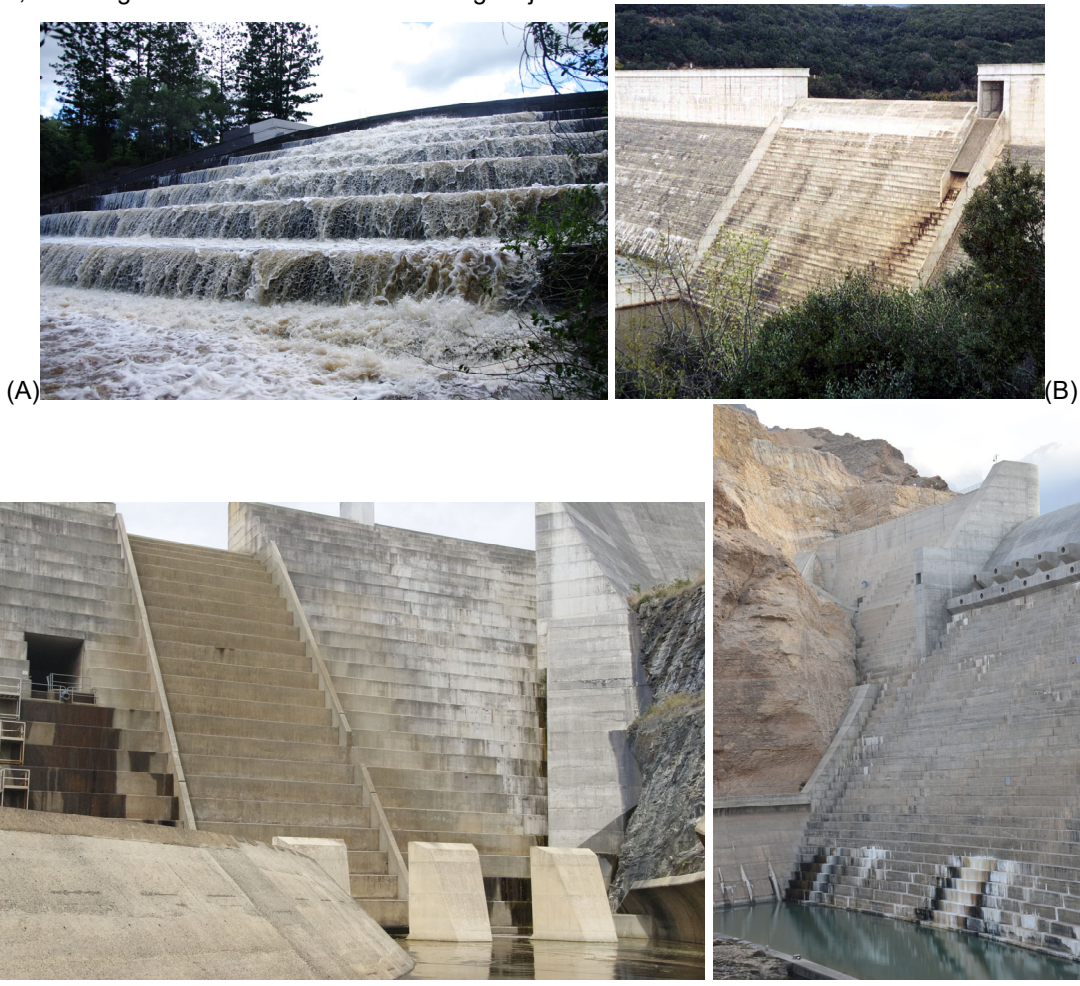
Figure 1. Stepped spillways. (A) Gold Creek Dam (Australia, 1890) on 23 February 2015; (B) Les Olivettes Dam (France, 1987) in March 2003 (Courtesy Mr & Mrs J. Chanson); (C) Hinze Dam Stage 3 (Australia, 2011) on 26 September 2018; (D) Wadi Dayqah Dam (Oman, 2012) in January 2018 (Courtesy Dr D. Wüthrich)
