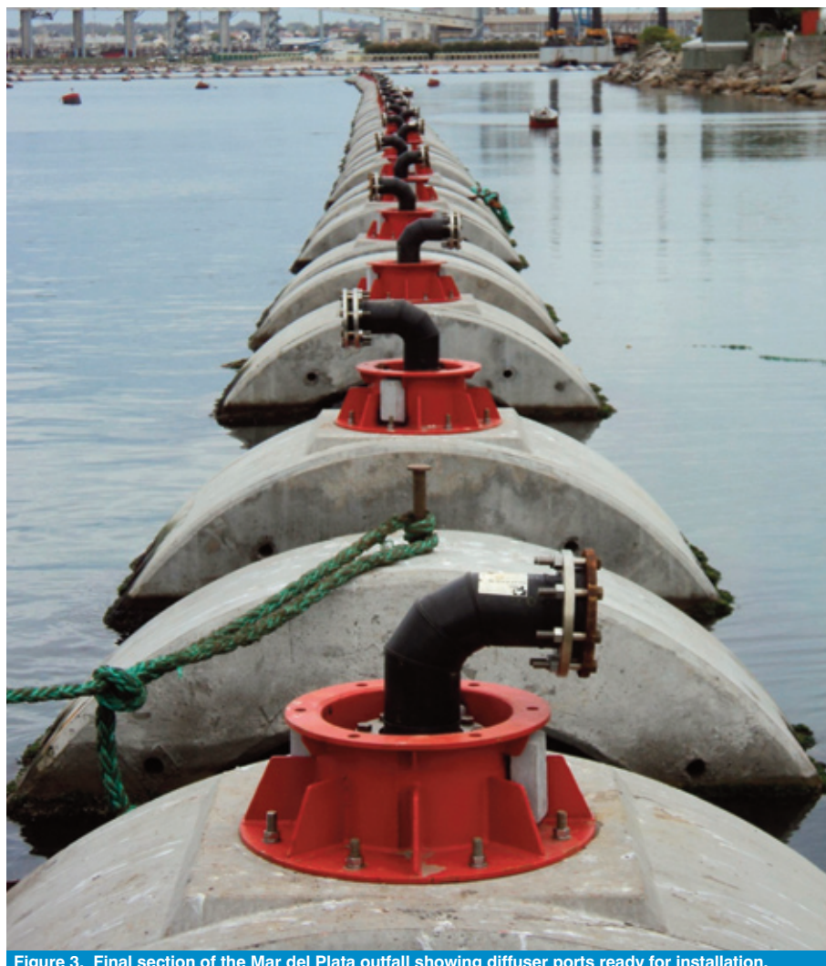
Figure 3. Final section of the Mar del Plata outfall showing diffuser ports ready for installation.
