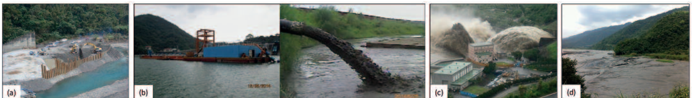
Figure 4. Sediment management strategies in Taiwan [5] : (a) mechanical dredging from a sabo dam in Yixing, Shihmen basin, (b) hydraulic dredging at Shihmen reservoir (photo courtesy of WRA), (c) Sluicing at Shihmen Reservoir during Typhoon Soulik in 2013 (WRA), (d) Drawdown flushing at Wujie Reservoir
