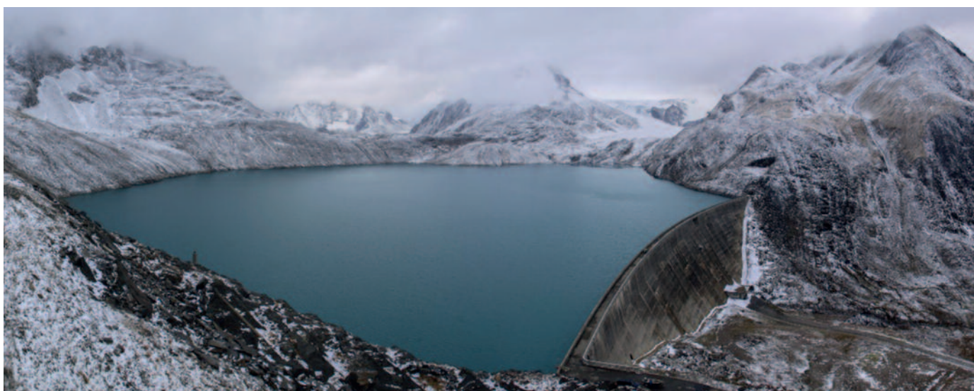
Figure 1. Griessee Reservoir with retreating glacier in the background, leading to higher sediment yield. (Photograph: D. Ehrbar, VAW, ETH Zurich)
