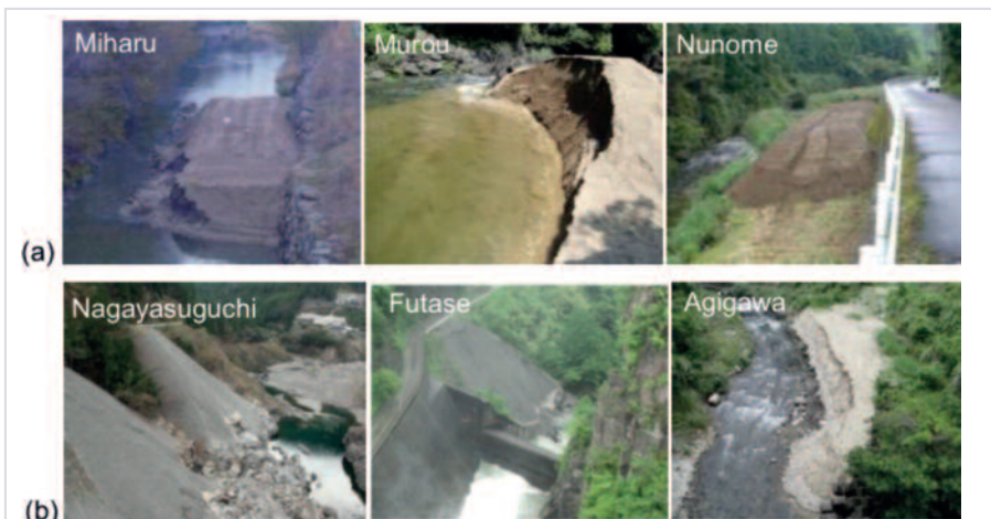
Figure 9. Sediment replenishment projects in Japan. (a) High-flow Stockpile, and (b) Point bar Stockpile
