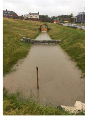
Figure 4: Swale under heavy rain conditions.
