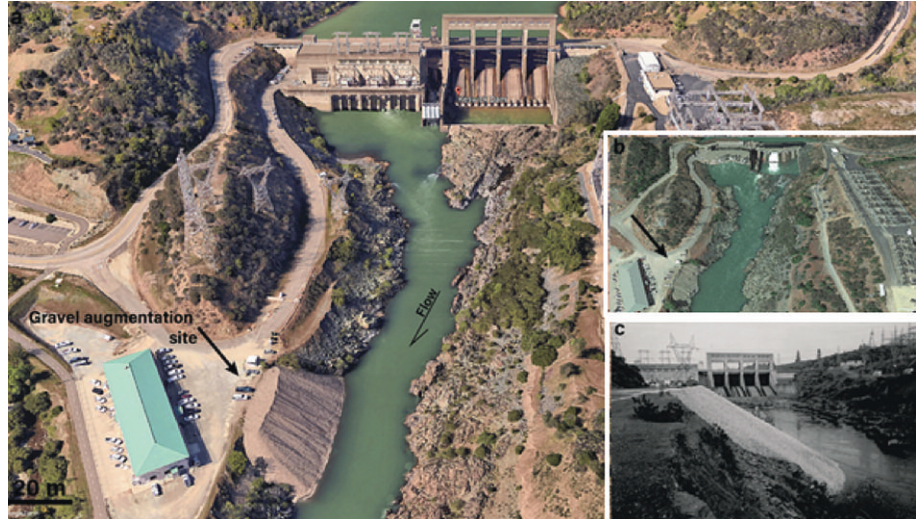
Figure 2. Gravel replenishment below Keswick Dam. To balance the sediment starvation created by trapping in Shasta and Keswick Dams, gravel is deposited from dump trucks down the bank of the Sacramento River, creating a cone to be eroded by subsequent high flows. (a) Remote-sensing composite image of site, showing gravel pile emplaced (15 April 2015), and (b) subsequently eroded (24 May 2017) (Google Earth). (c) Gravel augmentation has been ongoing here for decades, as reflected in a much-reproduced photo from January 1989 by Kondolf.
