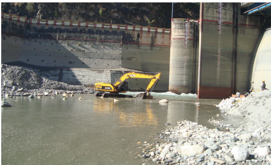
Figure 1. Sediment accumulation reduces storage volume and may interfere with the operation of dam outlet works. Removal of sediment by dredging or excavation (as shown in the photograph of the Maneri Bhalil Stage 1 dam during maintenance of the spillway.) may be needed to enable the dam to function.
