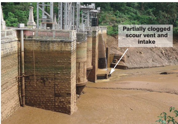
Figure 4. Sediment deposition at Kundah Palam in Tamil Nadu (left) and Maneri Bhali Stage-1 in Uttarakhand (right), revealing differences in source, feature and sedimentation rate
