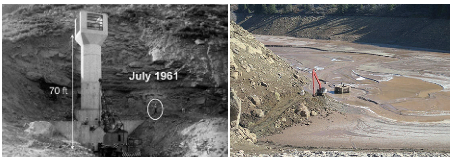
Figure 2. Paonia Reservoir near Hotchkiss, Colorado reached the end of its sediment design life after 50 years when the outlet became clogged with sediment and woody debris. The outlet was constructed in 1961, 21 m above the reservoir bottom (left). By 2014, the sediment level at the dam was 1 m higher than the outlet works (right). Photographs courtesy of Bureau of Reclamation
