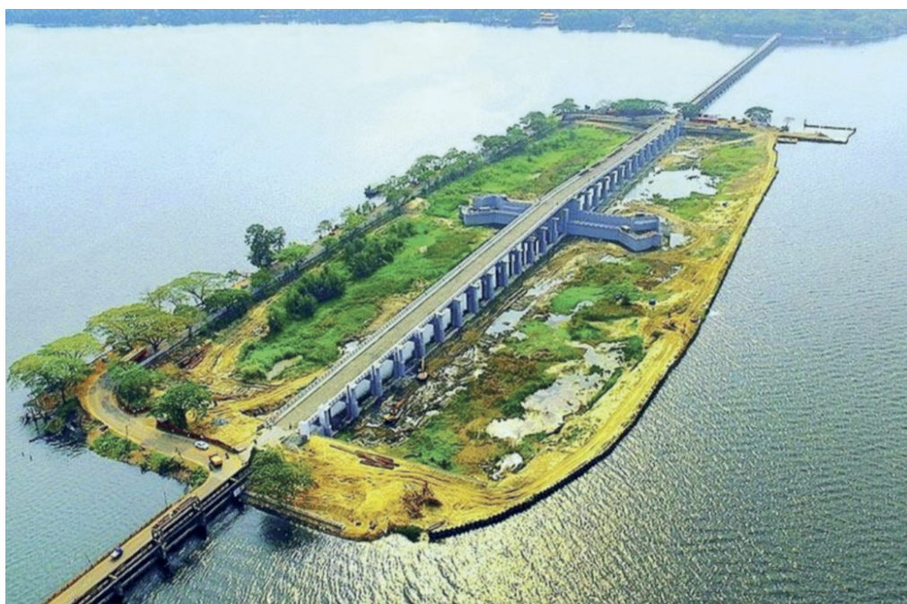
Figure 1. View of the Thaneermukkom bund
