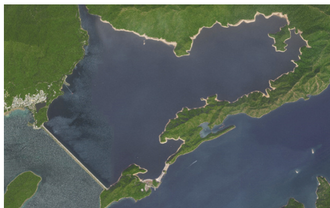
Figure 6. Aerial view of Plover Cove Reservoir
