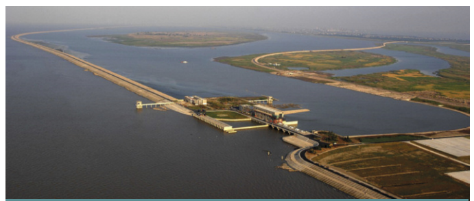
Figure 12. The water intake station of Qingcaosha Reservoir
