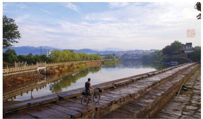
Figure 2. The Tuoshan Weir today
