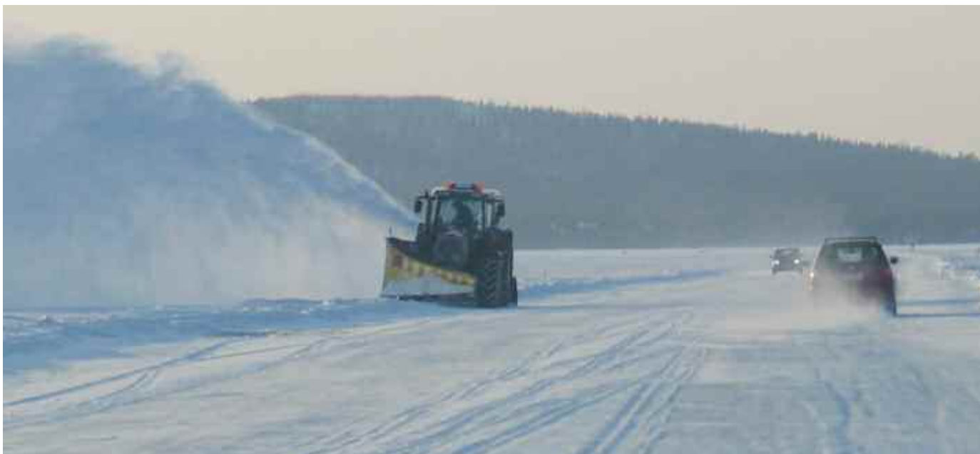
Figure 3. Ice road maintenance in Lake Pielinen, Finland. Photograph: Maritta Räsänen
