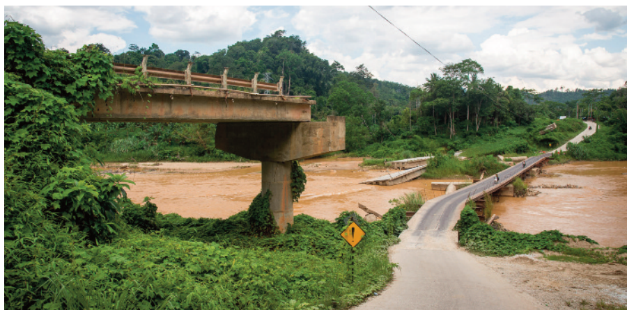
Figure 1. Extreme floods have caused significant damage to infrastructure in Malaysia. This bridge in Kelantan River was destroyed by the December 2014 flood
