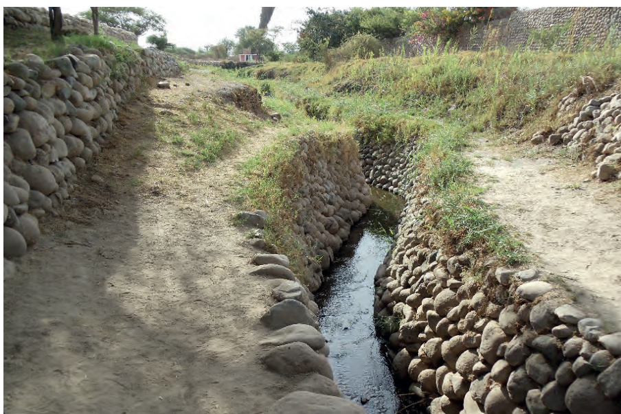
Figure 2. Cobble walls of Nazca canal downstream of filtration galleries. This irrigation structure is still in use
