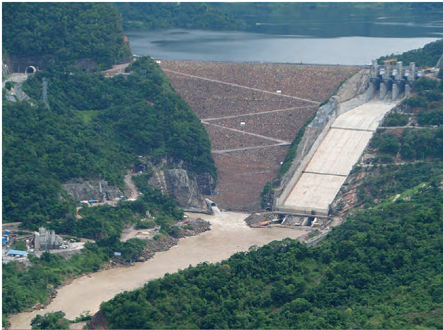
Figure 2. Sogamoso river Hydropower project, Magdalena-Cauca basin, Colombia
