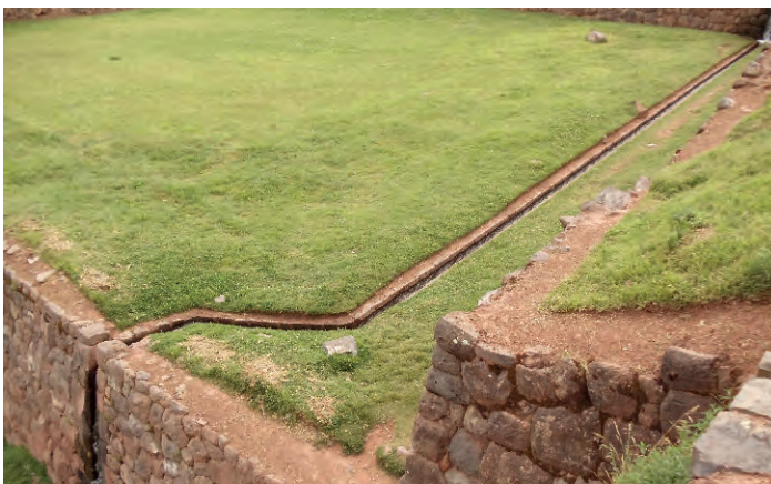
Figure 4. Rock canal and waterfall in Tipon, a small Inca urban center located 24 km South of Cusco City. Notice that energy losses are induced upstream of the waterfall by creating a sinuous path. Consequently, the jet trajectory stays close to the stone wall
