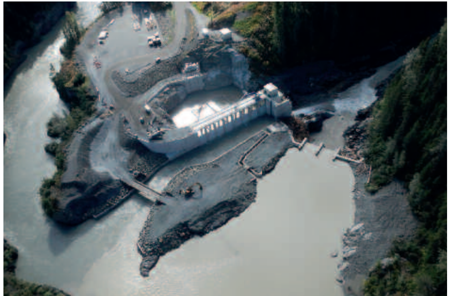
Figure 6 - Intake facility that includes field monitoring sensors, sediment sluicing facilities and a desander
