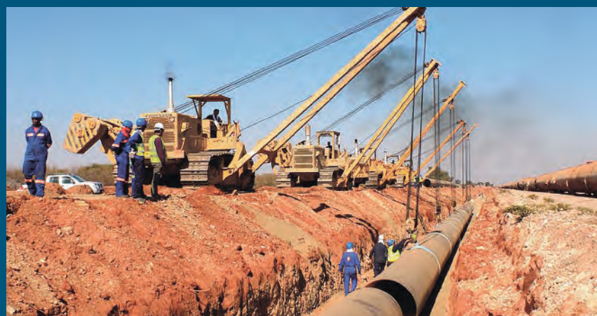
NSC Pipeline to convey water to Gaborone
