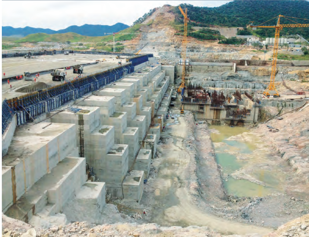
The Great Ethiopian Renaissance Dam project main dam view from the right abutment with the roller compacted concrete dam under construction, October 2014
