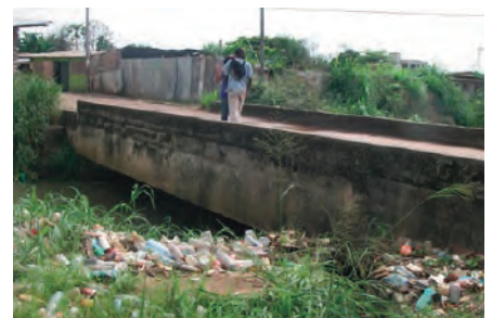
Figure 4 - Examples of severe hydraulic restrictions of flow under two bridges caused by the disposal of trash
