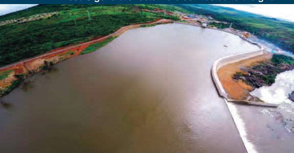
Panoramic view of KALETA Hydropower station, whose 3 generator sets were connected to the grid
