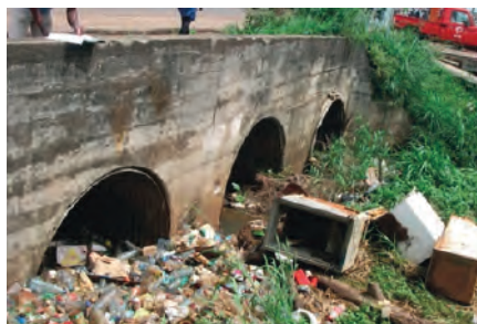
Figure 4 - Examples of severe hydraulic restrictions of flow under two bridges caused by the disposal of trash
