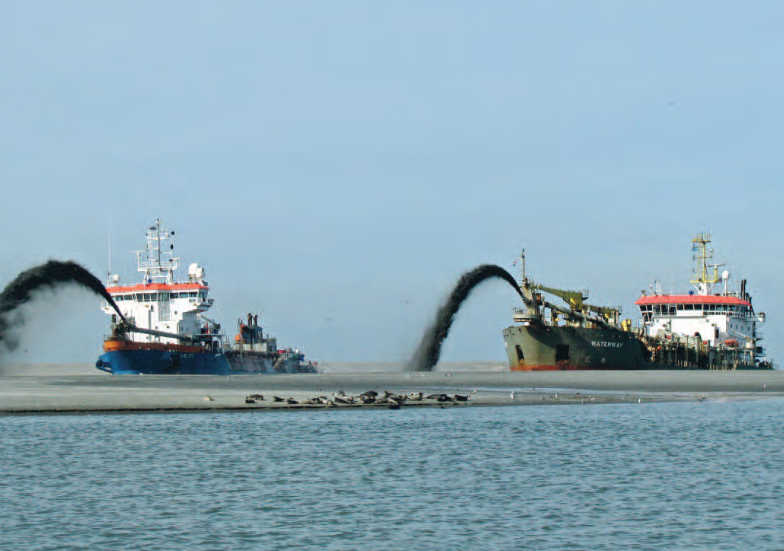
Hoppers of Van Oord (left) and Boskalis (right) working together in the construction of the Rotterdam Port Extension Maasvlakte II.
