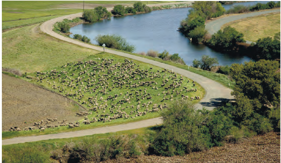
Subsided pasture lands on Twitchell Island, bordered by elevated Delta channel. Many levees throughout the Delta have a high probability of failure
