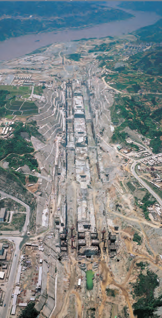
Dual-way Five-stage ship lock under excavation
