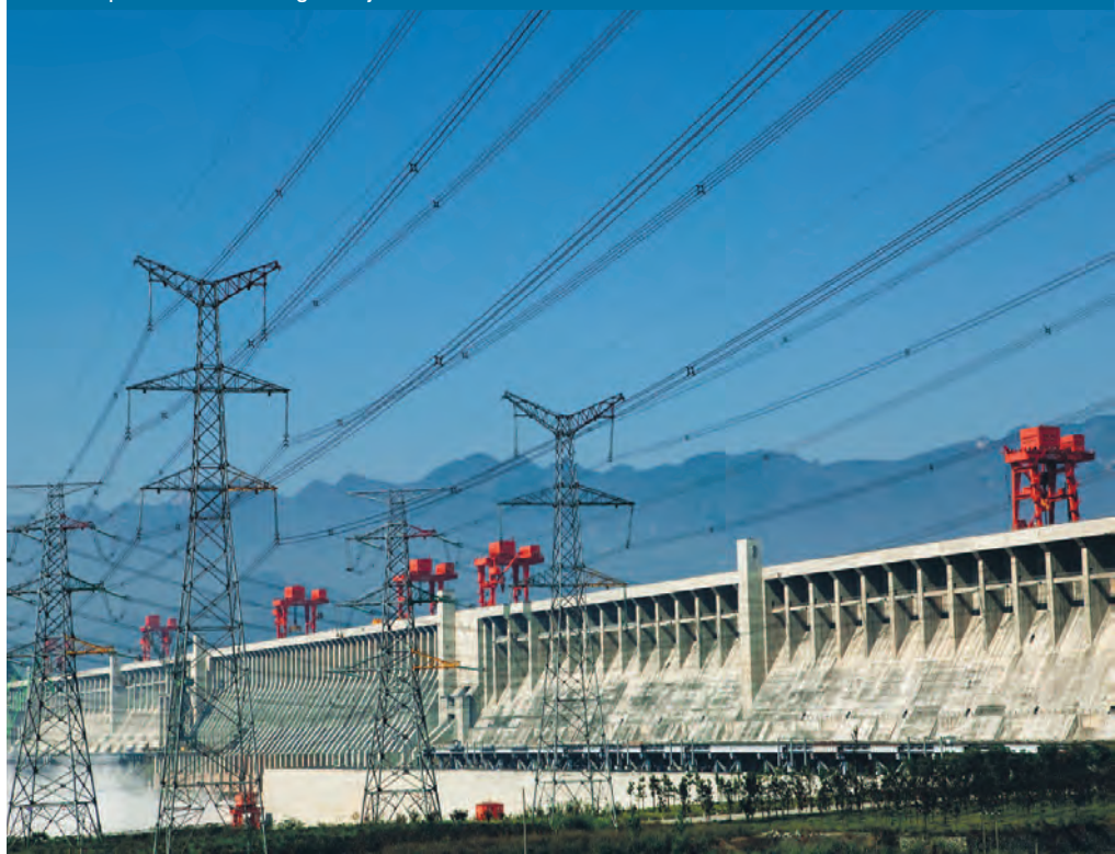
Power output of the Three Gorges Project
