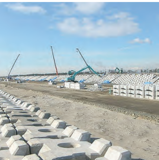
Fig. 1 Reconstruction of sea dyke along the Sendai Coast (Jan. 31, 2013, courtesy of Sendai Office of River and National Highway)
