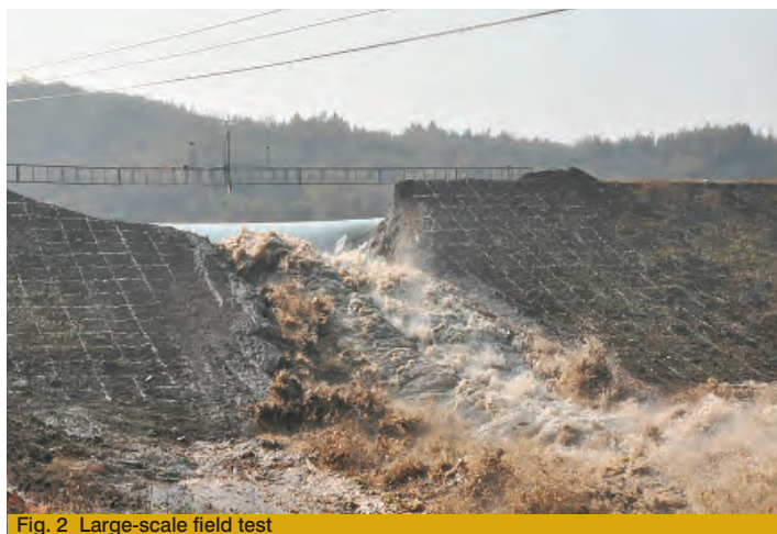
Fig. 2 Large-scale field test
