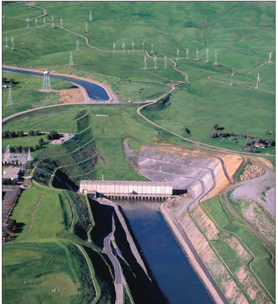
Figure 3. State Water Project's Harvey Banks Pumping Plant is powerful enough to alter circulation patterns in the Delta. The pumps also trap fish. Source: CA Dept of Water Resources.
