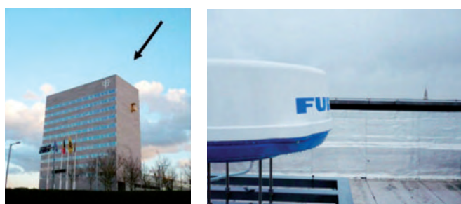
Fig. 2: Location of the Leuven X-band radar of Aquafin, on the roof of the Provinciehuis building.
