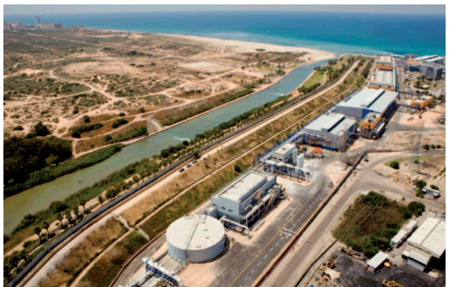
Hadera (Israel), world's largest RO desalination plant (275,000 m 3 /d, source: IDE Technologies)
