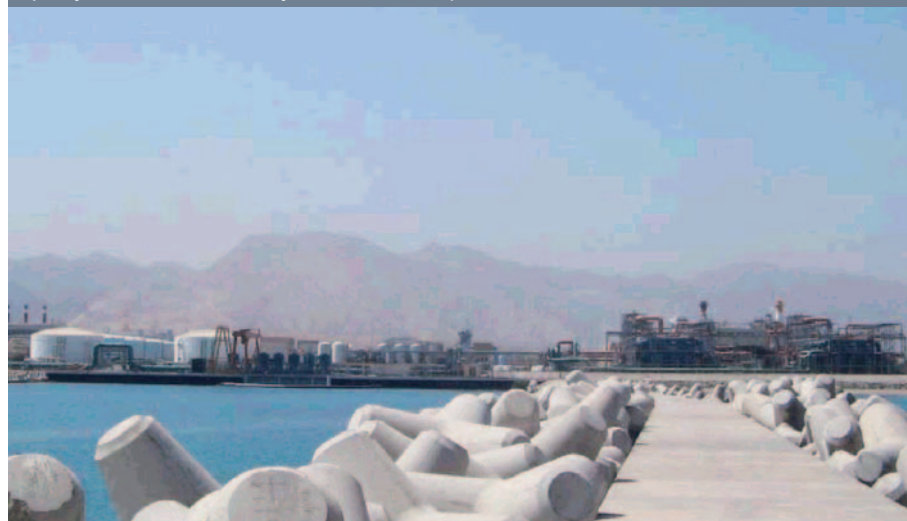
Muscat (Oman), Al Ghubrah power generation and seawater desalination plant (biggest in Oman, capacity: 191,000 m 3 /d, courtesy: HMR Consultants)
