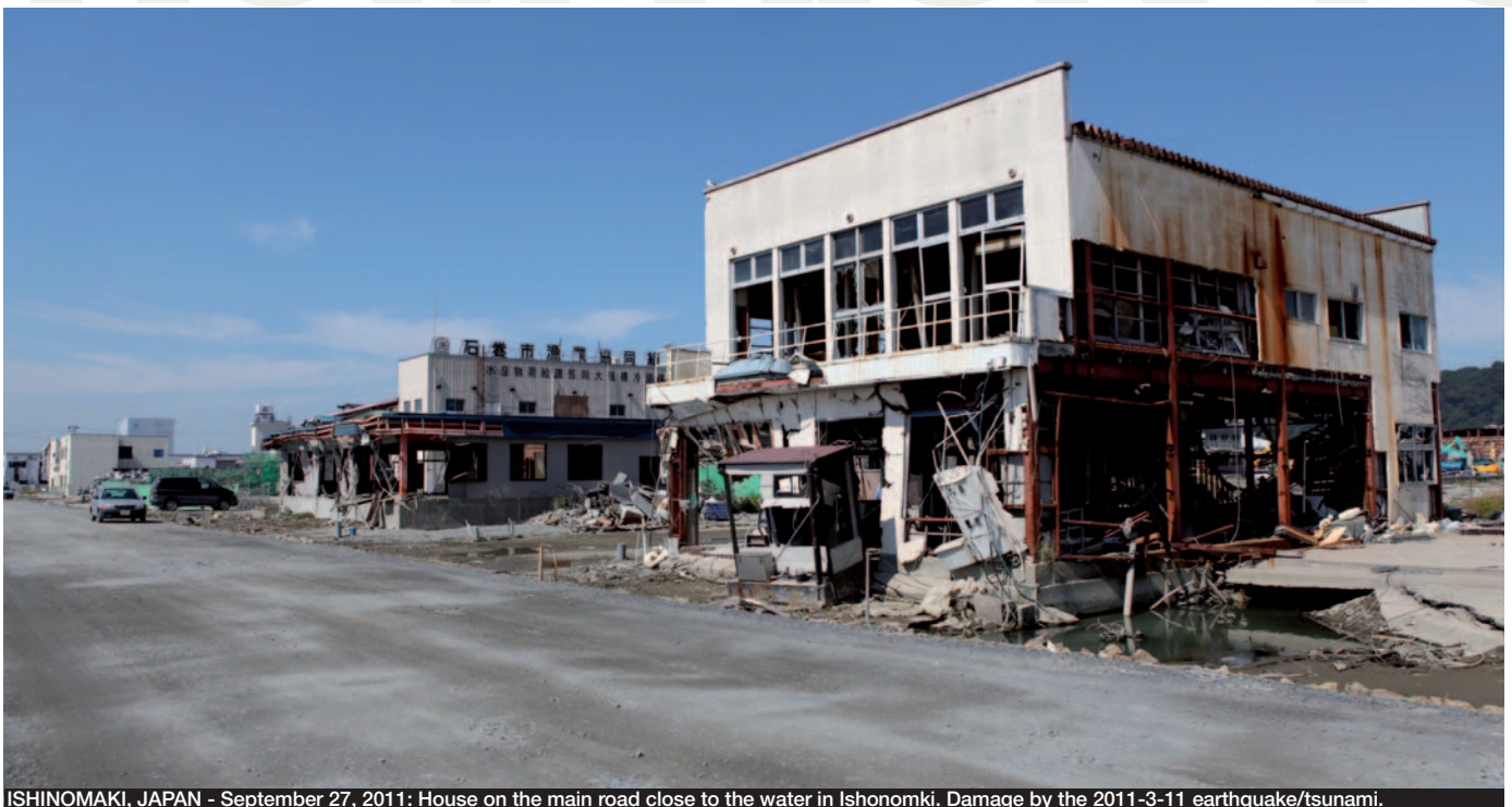
ISHINOMAKI, JAPAN - September 27, 2011: House on the main road close to the water in Ishinomaki. Damage by the 2011-3-11 earthquake/tsunami.
