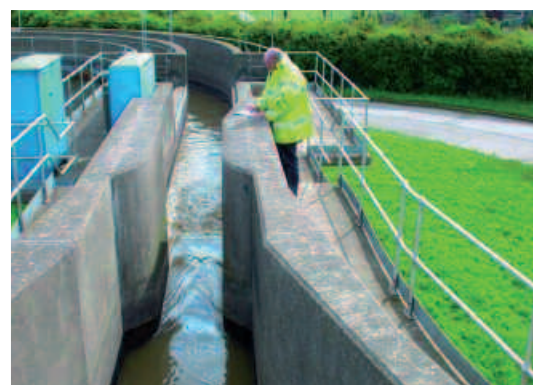
Figure 3 – Inspection of a flume on an effluent discharge channel to ensure compliance with the relevant flow measurement standards
