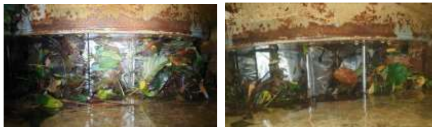
Figure 2. Visual inspections and accumulation of organic vegetal bodies: immediately after operation (left) and after few minutes of inactivity (right).
