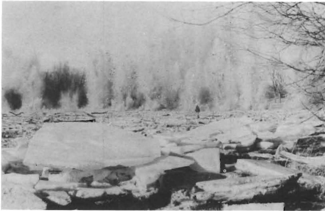
Figure 1. Blasting of ice jam on Iowa River near its confluence with Mississippi River, January, 1975.
