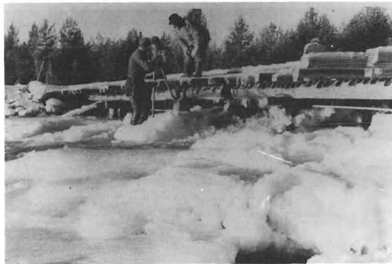
River Unsetåa, Øvre Rendal, 10. Dec. 1957. During 24 hours ca. 50 000 m 3 of sludge was accumulated on the front side of the bridge.
