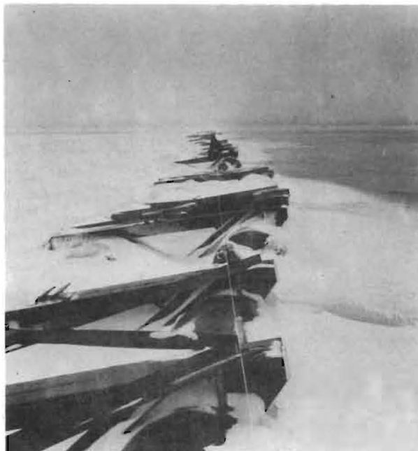
Figure 2. Loaded ice boom indicating sag of 118 ft (36 m) long section.
