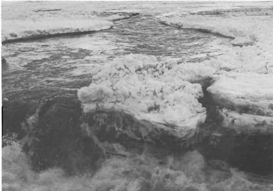
Fig. 6 Flow approaching through the rock jetty. Note the turbulent approach condition and the chunk of slush ice sitting on the ice skimming weir. Photo taken Nov. 13, 1970.
