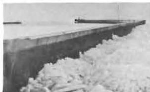
Fig. 8 Ice piling on the vertical breakwater at Hälsingborg, Sweden
