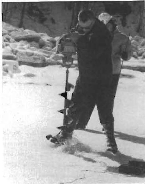
Figure 7. Drilling a placement hole with a power auger.
