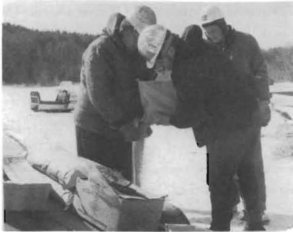
Figure 5. Transfer of the ANFO from its original container to a strong plastic bag.
