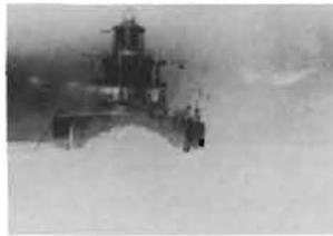
Fig. 3 Ice piling on Nordre Røse Lighthouse
