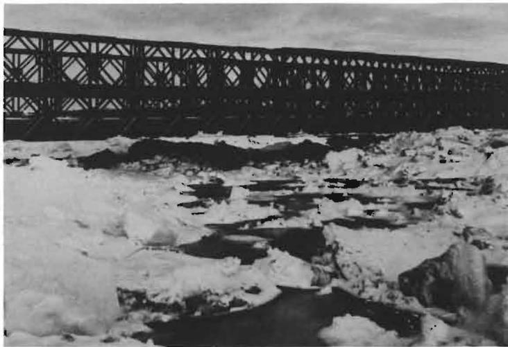
Fig. 5 Accumulation of pack-ice at Bailey bridge.
