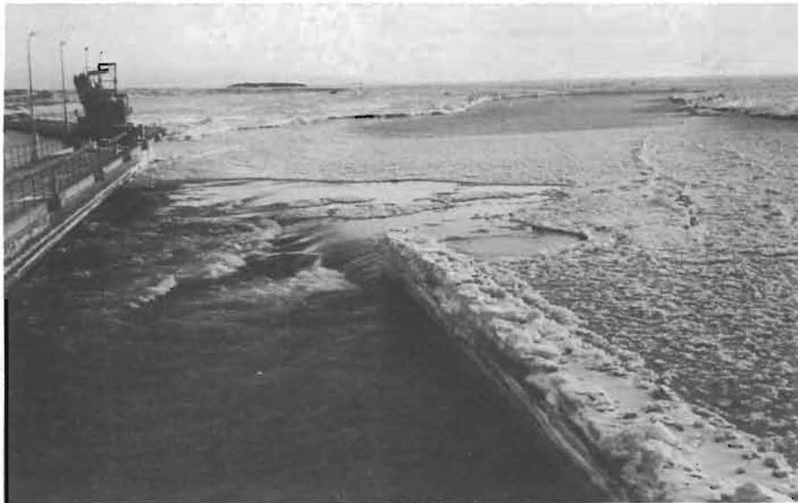
Fig. 7 Ice bridge about to form in front of the inlet.
