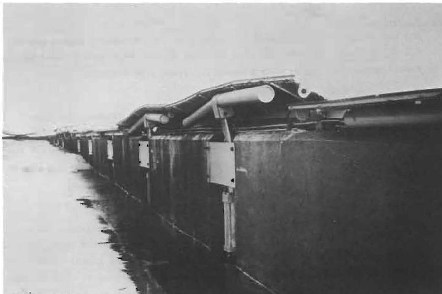
Fig. 9 The ice skimming weir on the apron wall in front of the ice sluice. The ice has destroyed this weir.
