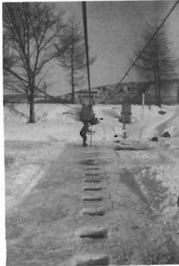
FIG.2 VELOCITY MEASUREMENT IN WINTERTIME AS PRACTISED ON HOKKAIDO, JAPAN.
