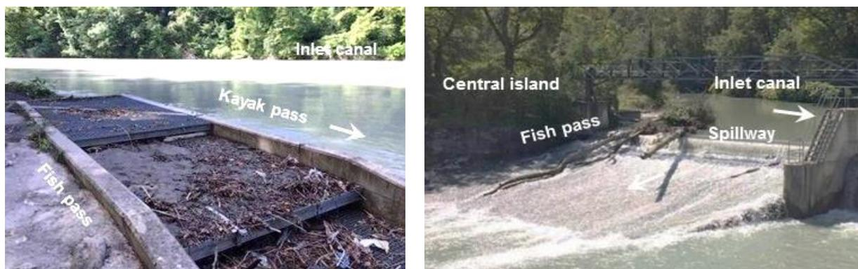
**Figure 3 Left:** Right-bank fish pass clogged by sand, silt and woody debris, due to floods milder than annual. **Right:** Central fish pass blocked by floated woods.
