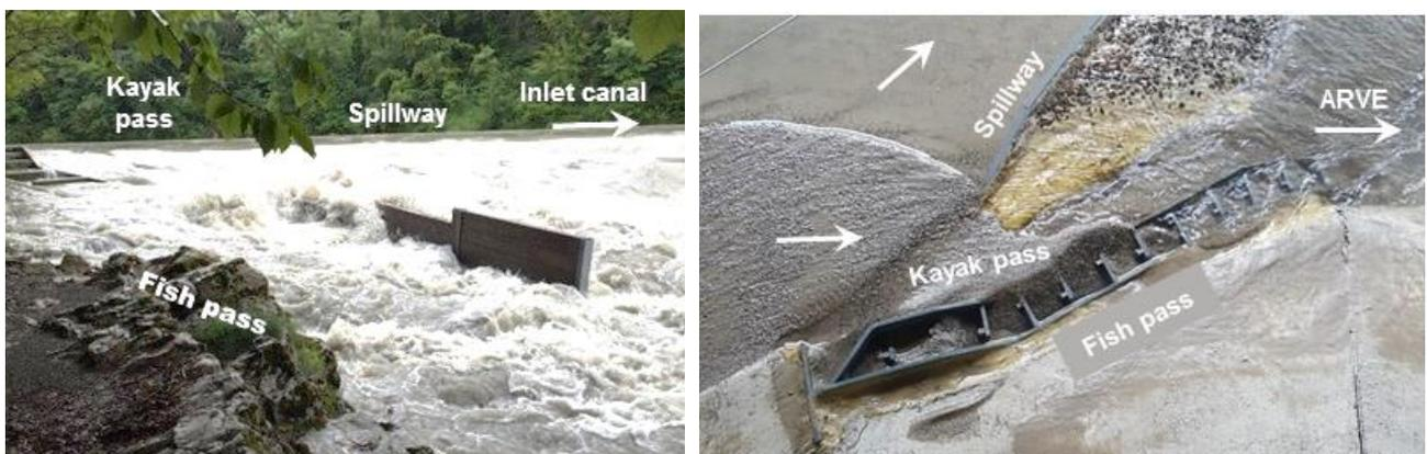
**Figure 14** The fish pass is overtopped by weak flow ( $T<1\text{y}$ ) of Arve, making its entrance inoperative. Bed load deposit upstream from the fish pass and fills up all compartments. Left: Arve River. Right: physical model.
